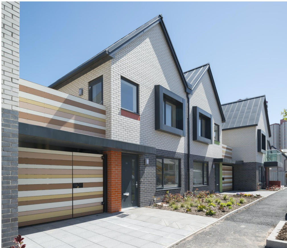
Above: Affordable housing at Queens Park, Blackpool
